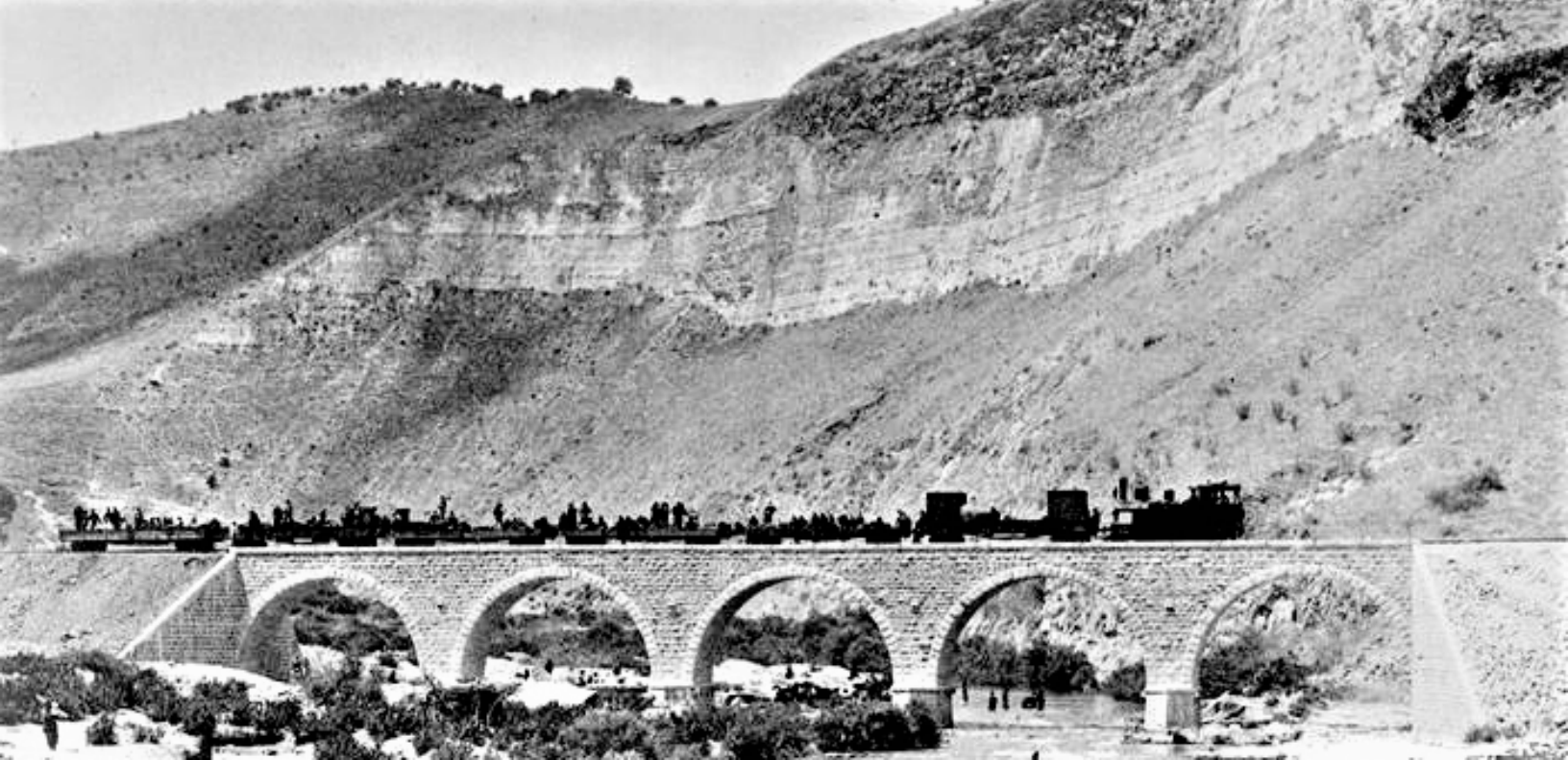
Hejaz Railway stone viaduct near Makarim, 1908 – Unknown author, public domain
